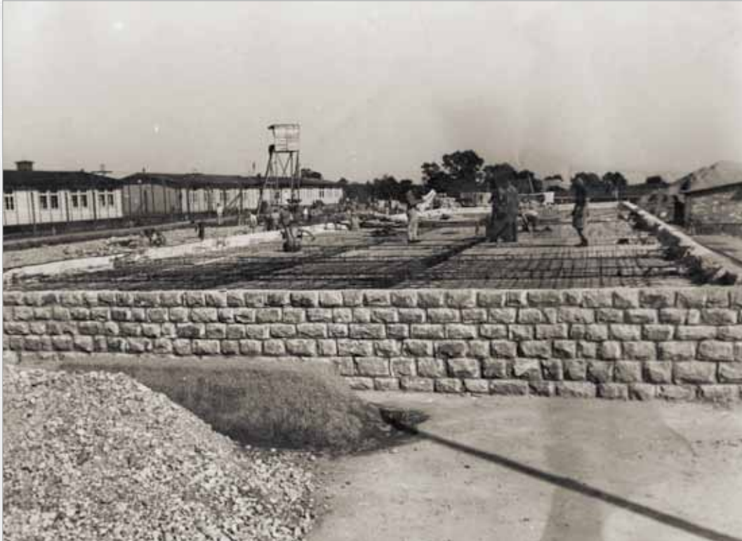
Above: Construction site of the infirmary building, circa 1941. The steel reinforcement of the basement ceiling is clearly visible (© Photograph Archive of the Mauthausen Memorial, L'Humanité Collection).
