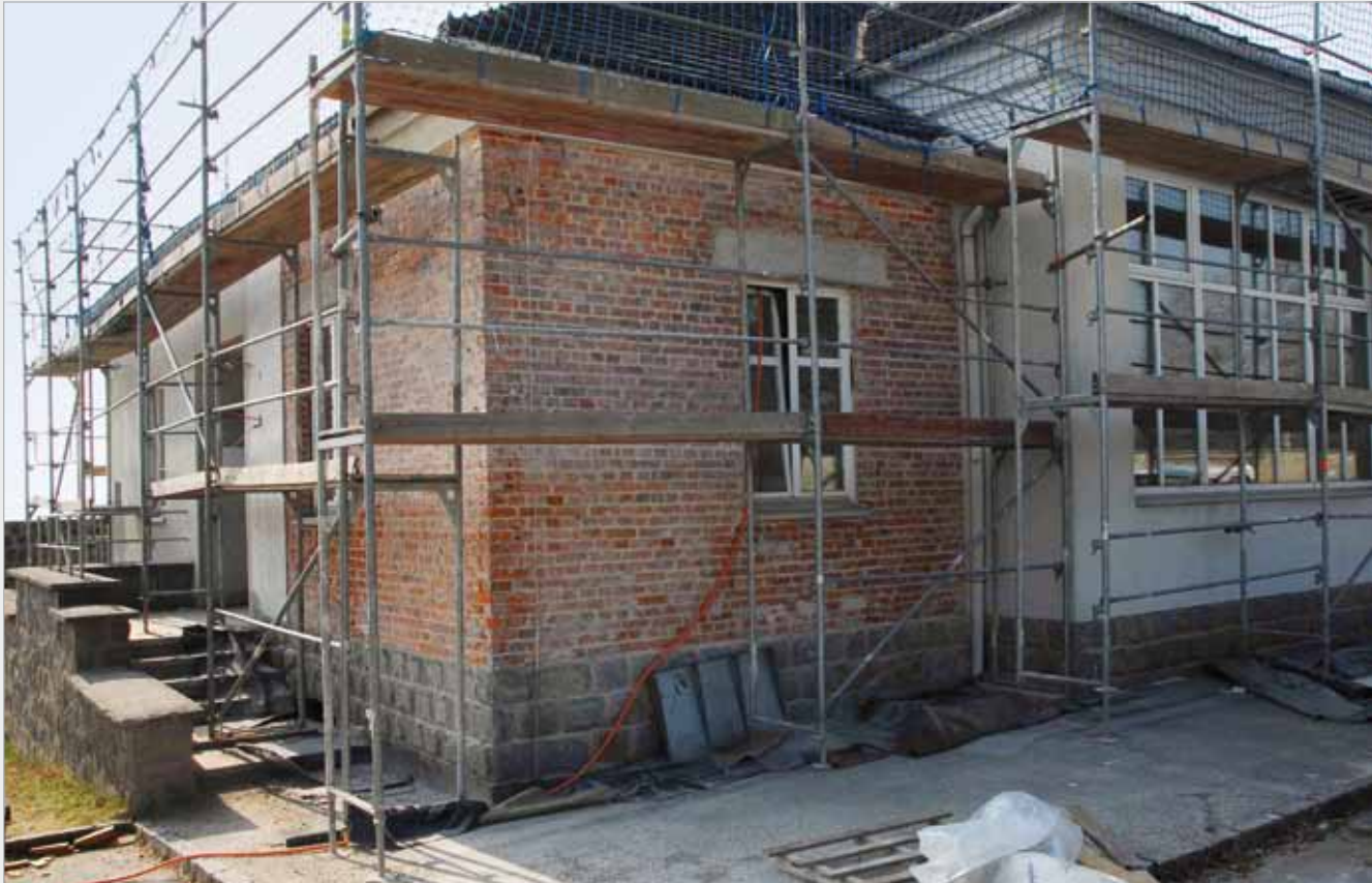
Facade of the former infirmary building in scaffolding during renovations; the building is being used as a museum. The section of the building without plastering functions as a 'historical window' onto how it looked in 1945 (© Federal Ministry of the Interior/Stephan Matyus).
